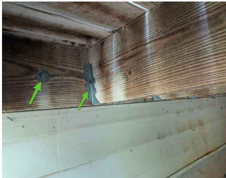
Ledge Bolted to the house framing Joist hangers w/ Proper nails
