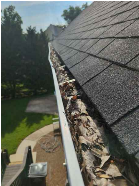
Rear Gutter System
