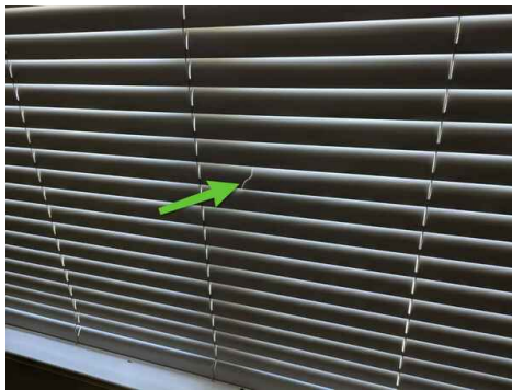
Blind has a crack in it.
