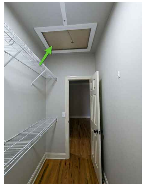
Attic Access Located in master bedroom closet
