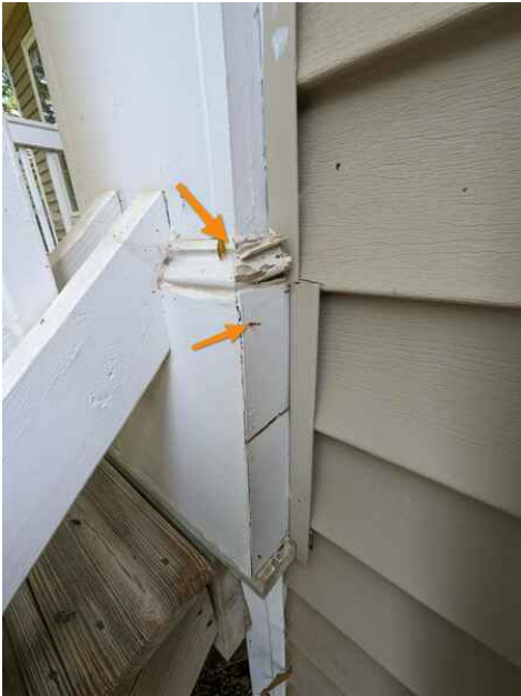
Moisture damaged wood and a loose trim nail show signs of previous water intrusion.
