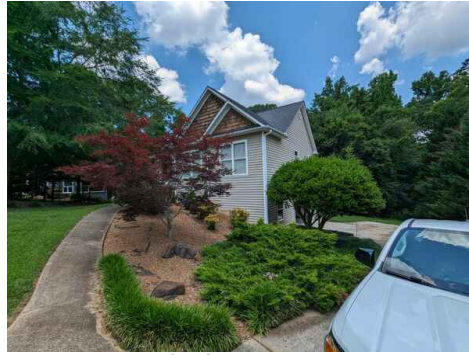
Right front Corner
