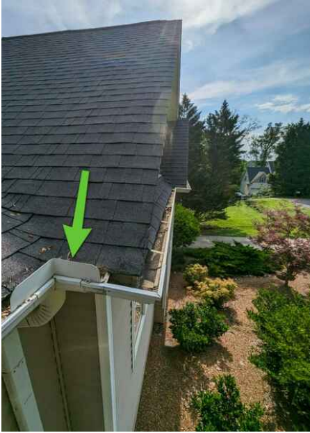
Kick-out flashing front valley porch side
