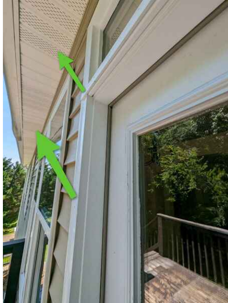
Soffit Venting
